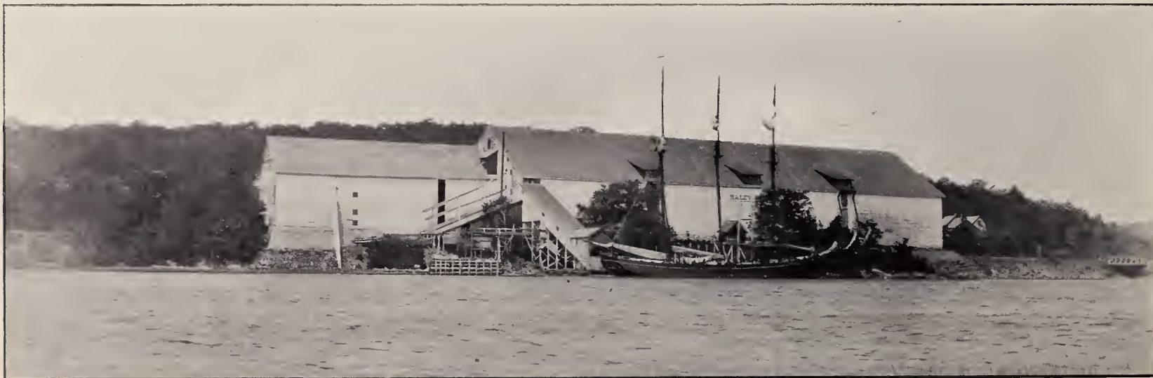
VIEW OF E. D. HALEY'S ICE PLANT.
